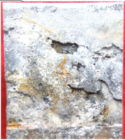
(a) cracked surface of aluminium alloy
